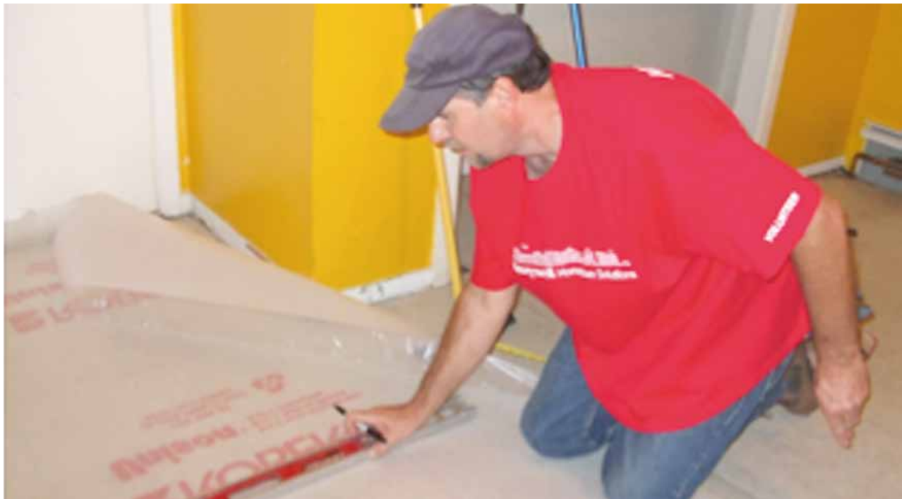
Carl Hitta of the Honeywell Corporation works on a RTLI project.
